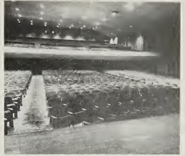
The Lee's auditorium, as seen from the rear, left, and from the stage, above, has a California stucco ceiling, upper walls of acoustical masonite, and lower walls of oak paneling. The simple lines are reminiscent of modern European design.
